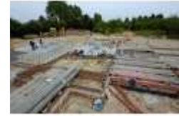
Block and Beam Flooring Method Statement
