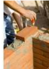
General Brick and Block Work Method Statement
