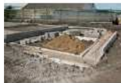
Concrete Foundations Method Statement
